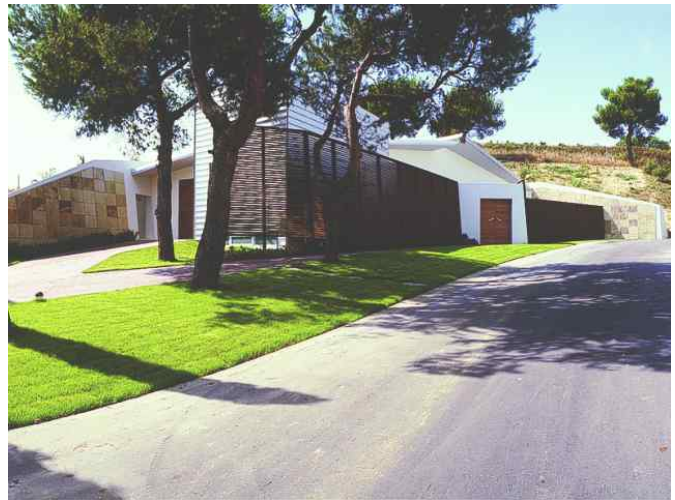
Outside view of the room for the aging of Umani Ronchi's wines
